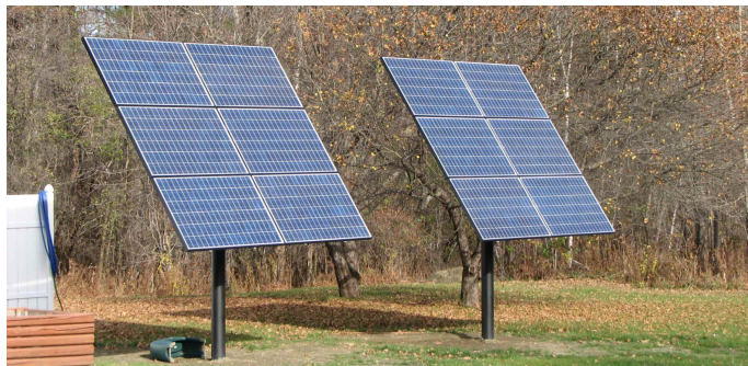
Figure 4: Pole Ground Mounted Solar Panels
